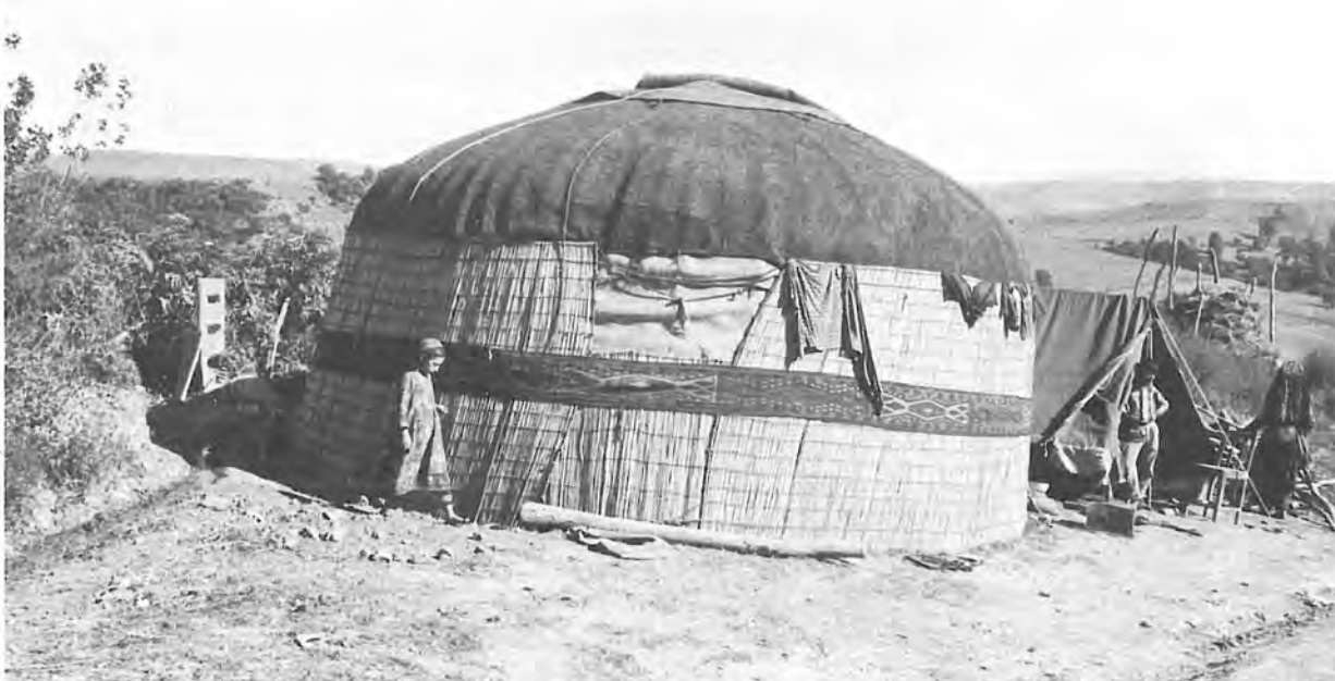
Plate 3. Turkoman yurt in northeastern Iran after the destructive earthquake of 30 July 1970.
