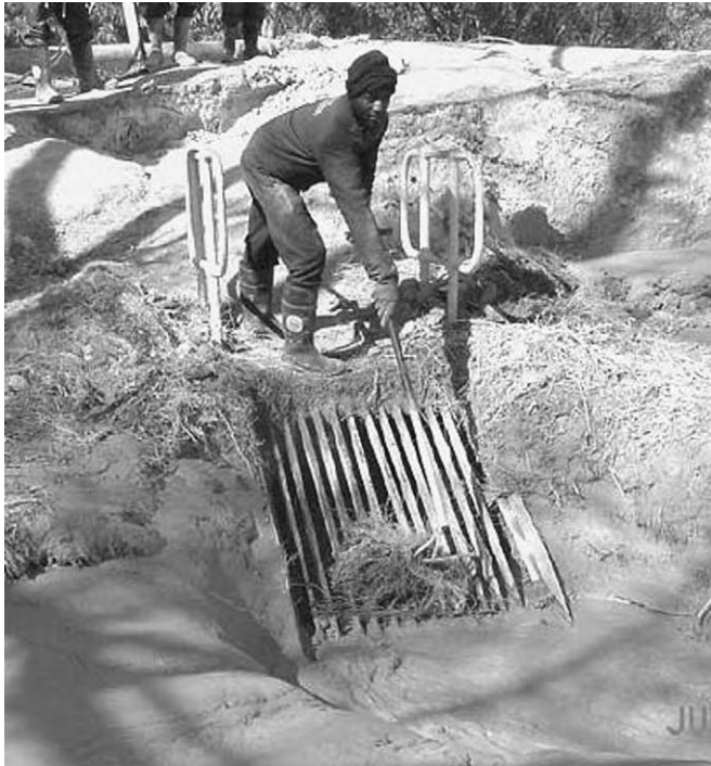
Fig. 4. Finger screen installation.
