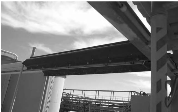
Fig. 8. Secondary containment for pipelines.
