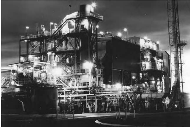
Fig. 4. Kanowna Belle roaster and arsenic bag-filter.
