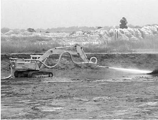
Fig. 1. Excavator-mounted monitor gun.
