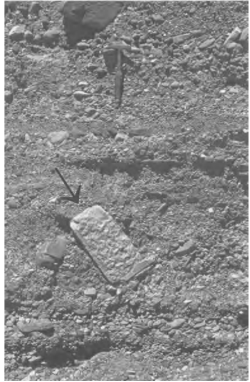
Fig. 19. Terrace T_1 of the Albarracín (A in Fig. 5) telescopic-like alluvial fan contains (arrow) a man-made (ashlar) block, the remnant of an old bridge of the N 20 national road, which collapsed due to natural causes between 1968 and 1972.
