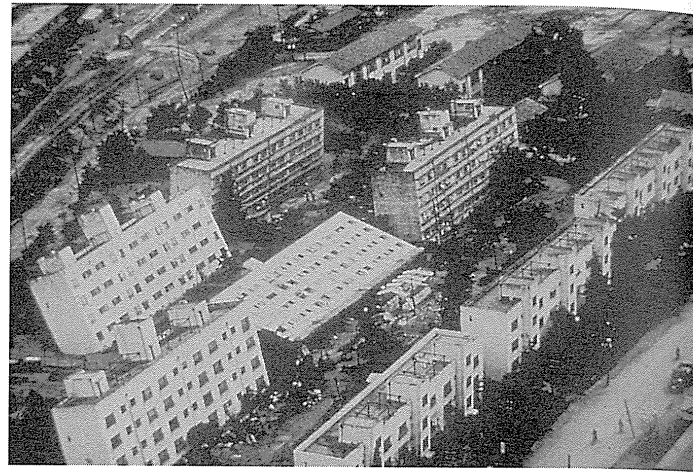
Fig. 1.2-13 Damage to apartment buildings caused by soil liquefaction during the June 16, 1964, Niigata (Japan) earthquake. About a third of the city sank by as much as 2 m as a result of sand compaction. (Courtesy of the National Geophysical Data Center.)
