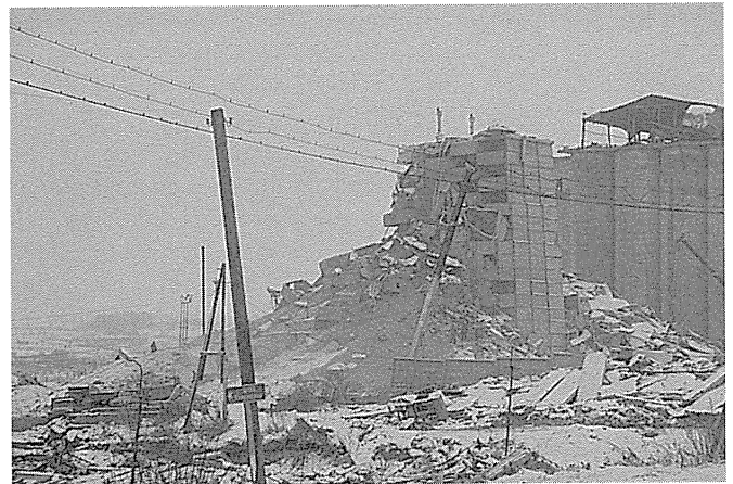
Fig. 1.2-7 Five-story building in Spitak, Armenia, destroyed during the December 7, 1988, earthquake. The building was made from precast concrete frames that were inadequately connected. The failure of such buildings contributed greatly to the loss of 25,000 lives. (Courtesy of the US Geological Survey.)
